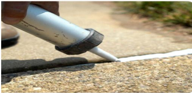
Sealing Construction Joint
