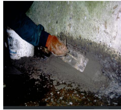
Fill floor cracks or add fillet between floor and wall
