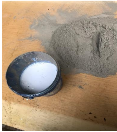
Mix slurry paste with SBR
