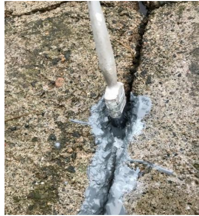
Paint slurry paste on crack edges
