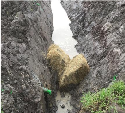
Hay bale sediment trap. Photo Source: Aqualinc
