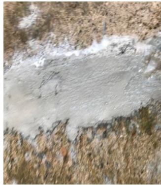
Fill floor cracks or add fillet between floor and wall
