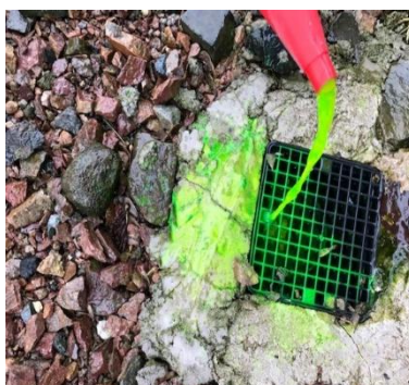
Drain tracing using non-toxic fluorescent dye
