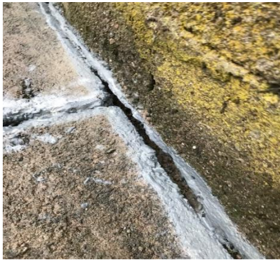
Apply repair mix before slurry dries
